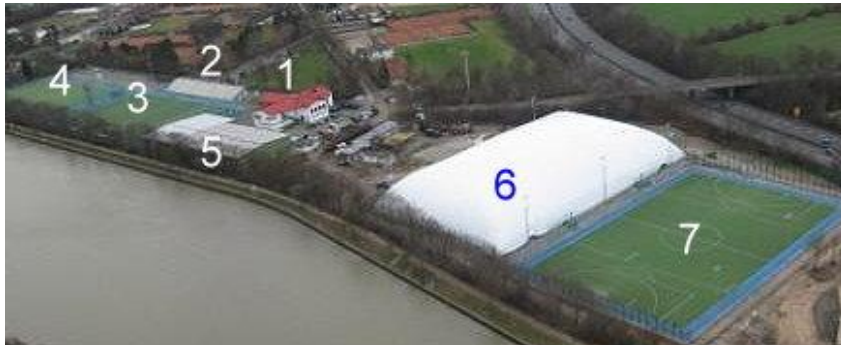
Mannheim Club Facilities – Several Fields
